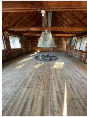
Jr House Improvements
